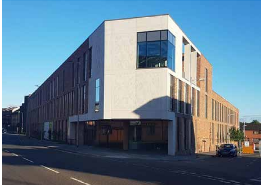
Pictured: The new Woodside Health and Care Centre.
