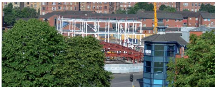
Site construction images
