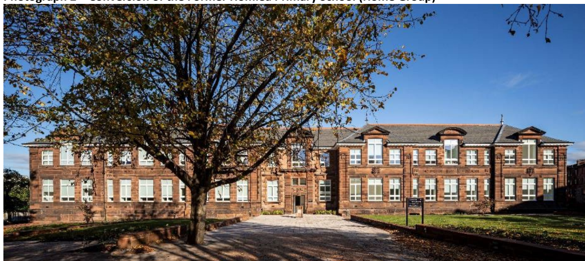
Photograph 2 – Conversion of the Former Homlea Primary School (Home Group) 2
