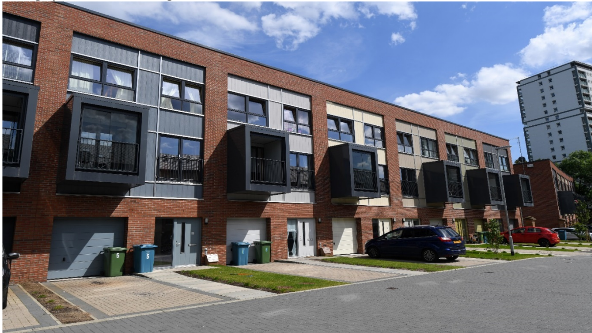
Photograph 1 – Partick Housing Association Broomlea
