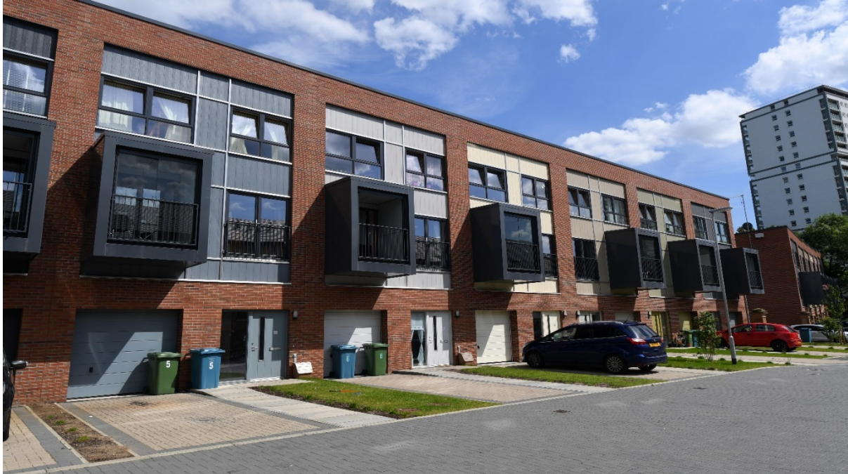
Photograph 1 – Partick Housing Association Broomlea
